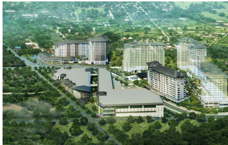
SERIN EAST TOWER 4 PHASE 2 (MAR) Tagaytay City, Cavite 413 units, P2.8B | 10% take-up
