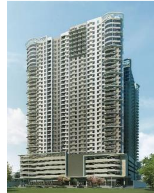
Towers Asten 3 (Mar 2017) Makati, Metro Manila 863 units, P3.7B 45% take-up
