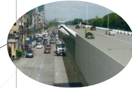
UP Town Center-Ateneo Viaduct 2017
